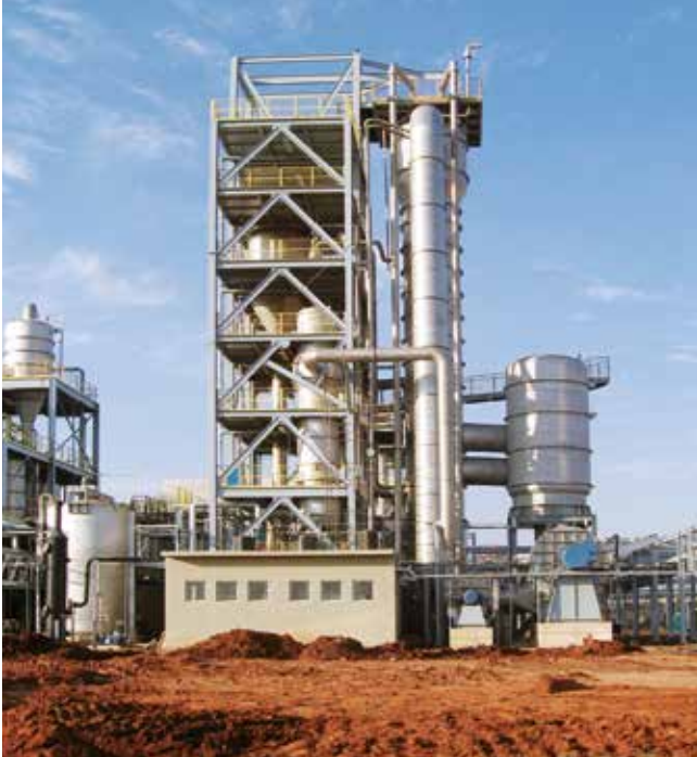
Evaporation plant with two fans for mechanical vapor recompression and forced circulation as finisher. Evaporation rate: 67 t/h
