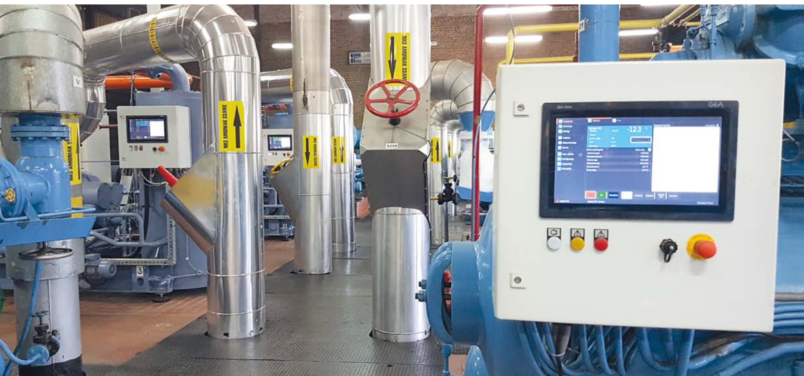
Below: A GEA Omni retrofit panel installed on a non-GEA compressor package (foreground) has the same appearance and functions as GEA Omni panels supplied on standard GEA compressor packages (background, left).
